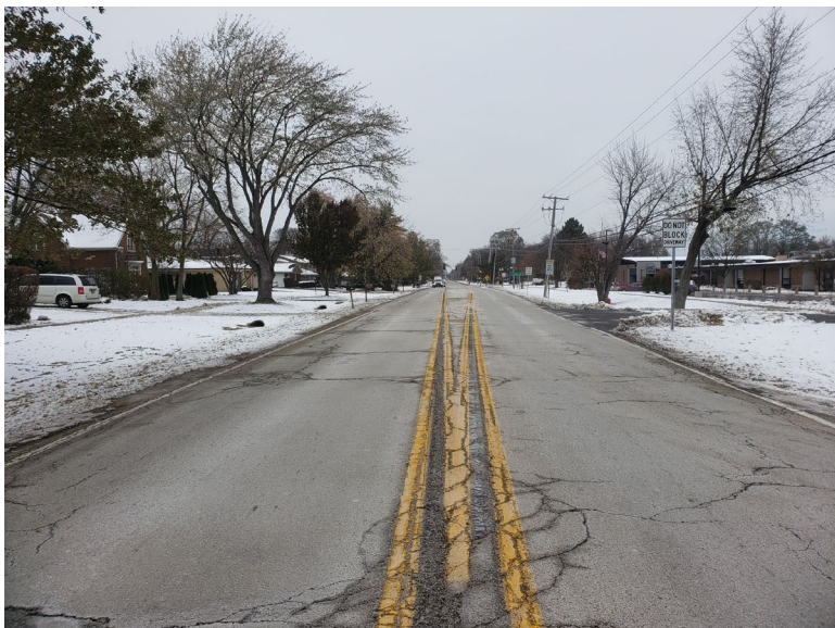
Northbound Landwehr Rd (South school access drive intersection)
