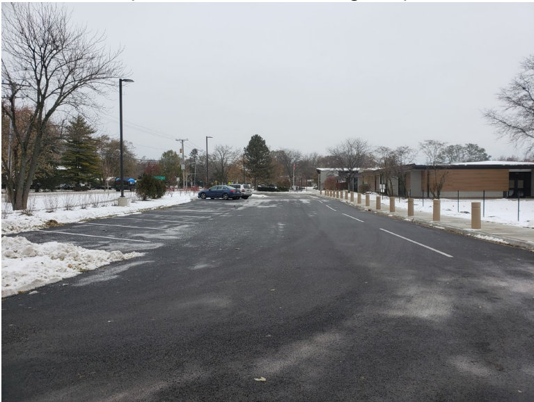
School access drive (off Landwehr Rd, facing North)
