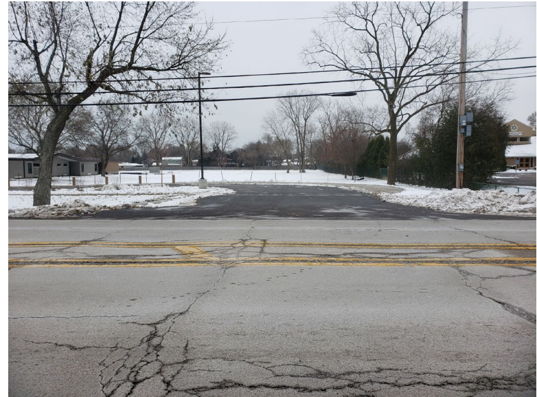
South school access drive (from Landwehr Rd, facing East)
