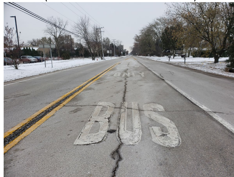
Southbound Landwehr Rd (between school access drives)
